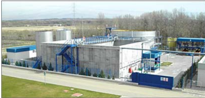
Pfizer Algete facility's wastewater treatment plant
