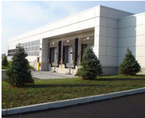
A solar panel roof on Building 98 at the Groton, Conn. campus generates energy equivalent to more than 10,000 barrels of oil each year.
